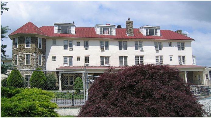
Abandoned/condemned Hill Top Inn
