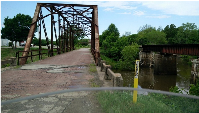
Another old 66 bridge, west of Tulsa, OK
