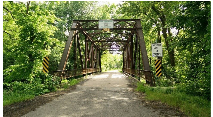
The Pryor Creek Route 66 Bridge
